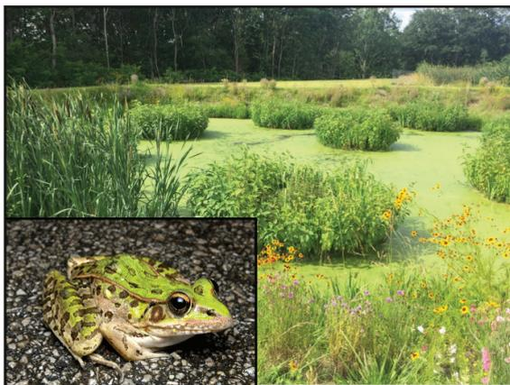
FIGURE 1. Treated effluent moves through three consecutive cells of a constructed wetland (CW) complex planted with native vegetation and colonized by native wildlife such as the Southern Leopard Frog (*Lithobates sphenoccephalus*; inset) observed in this study at Sewanee, Tennessee, USA. The shallow second cell of the wastewater treatment CW is pictured here. (Photographed by Saunders Drukker).
